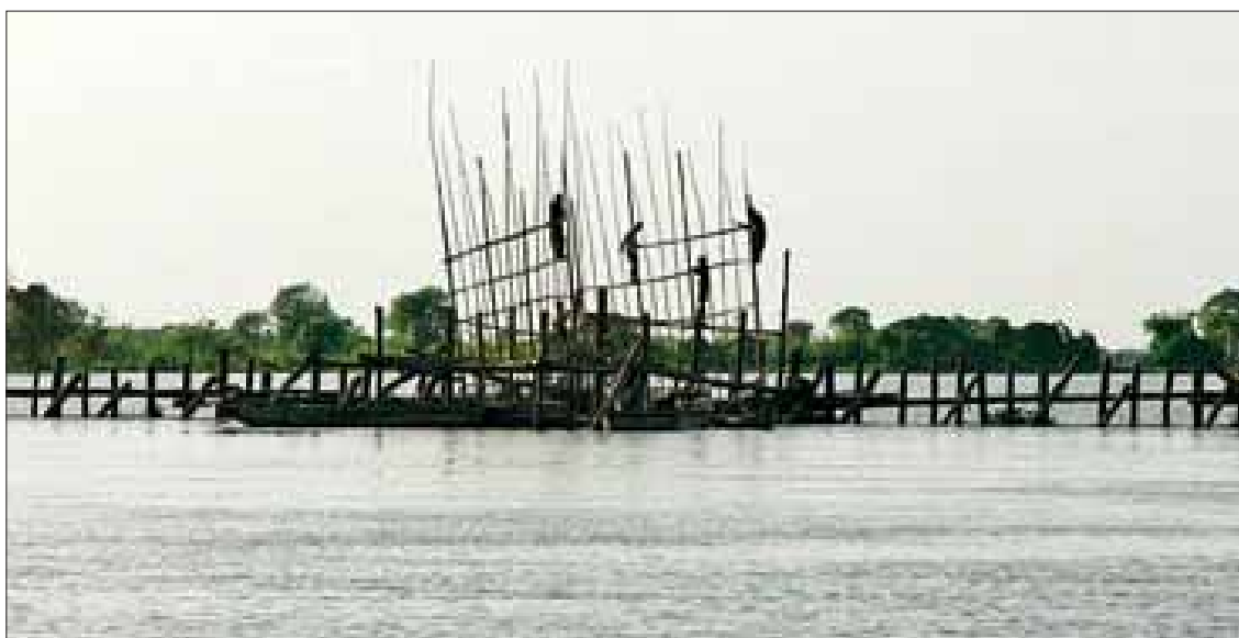
Figure 17: Construction of a fishing lot barrage in the Tonle Sap River.
